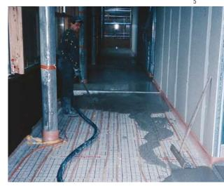
With the appropriate worm parts, you can even pump self levelling floor screed easily and economically
