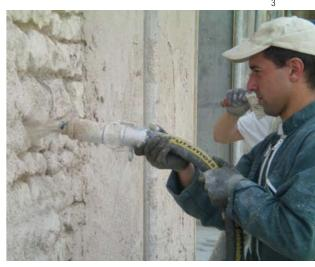
SP 11 worm pumps can be used inside and out for all site-made mixes and premixed dry mortar up to 6 mm.
