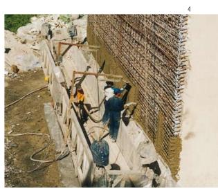
They are also extremely suitable for large jobs, as here for the concrete refurbishment of a motorway bridge in Italy.
